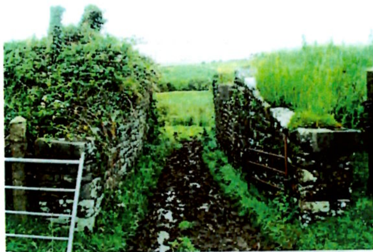
Photograph 10 Bridge removed at Cattle Crossing
