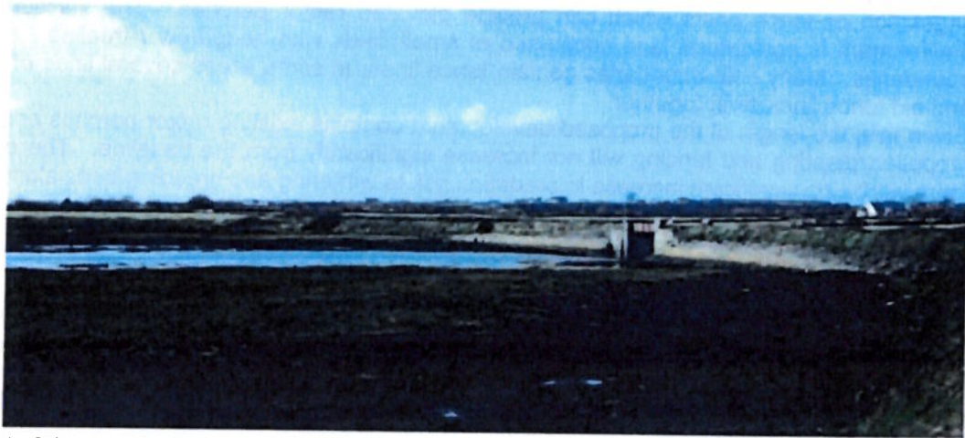
Plate 2.3 Moyasta bridge and causeway at low tide
