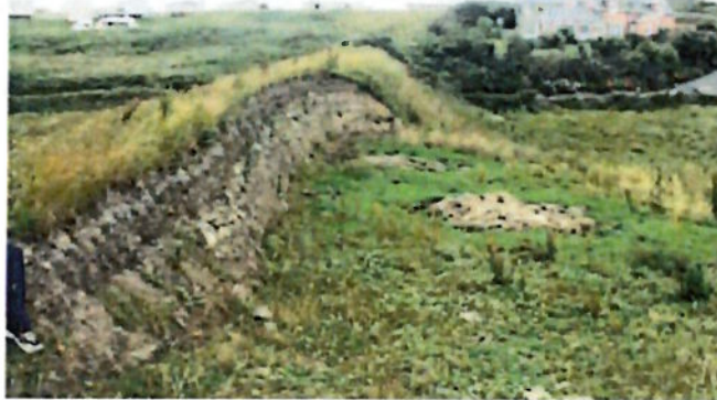
Photograph 9 Embankment partially removed
