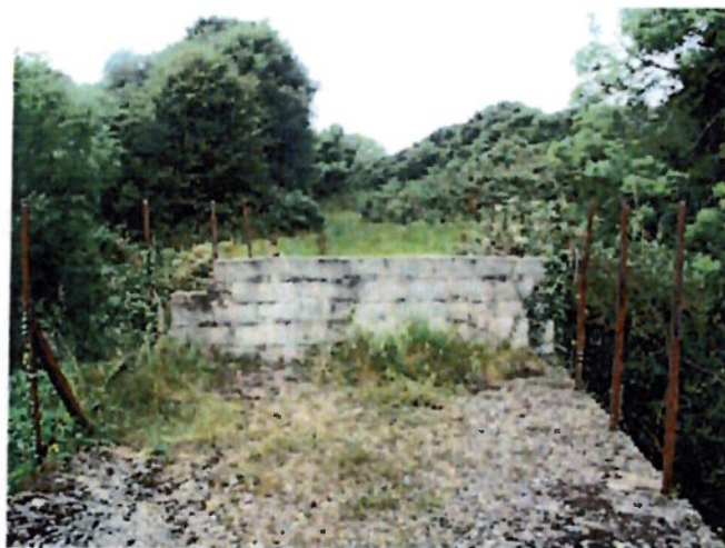
Photograph 6 Wall across bridge at Ennistymon
